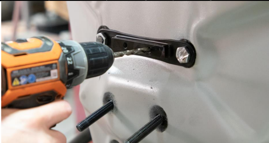
Figure 8: Drill into frame using brace plate as a guide.
