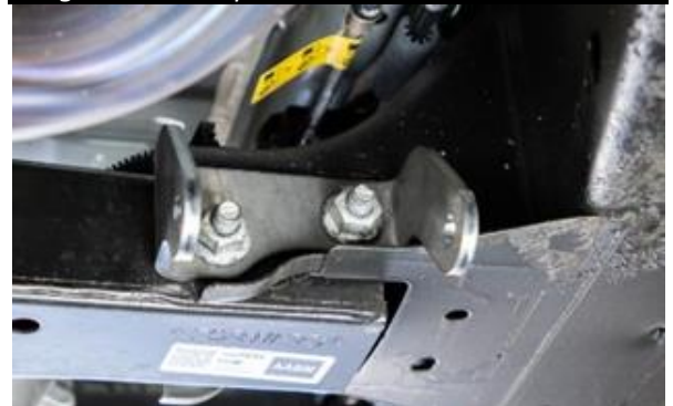
Figure 64: Compression Strut Mount Installed.
