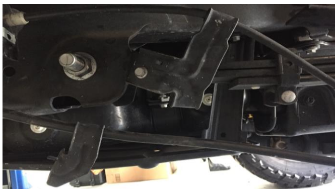
Figure 3: Brake Cable Removed
