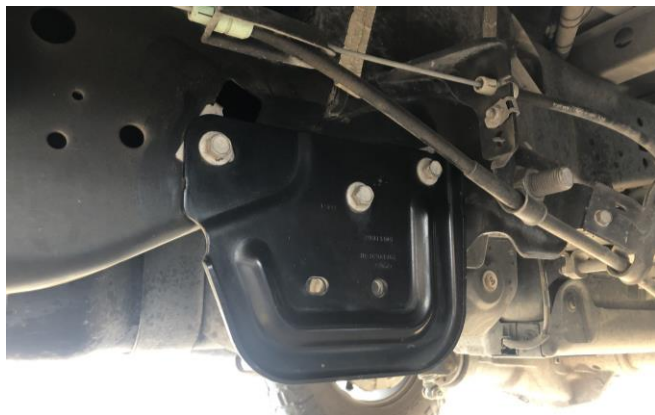
Figure 1: Fuel Tank Stone Deflector
