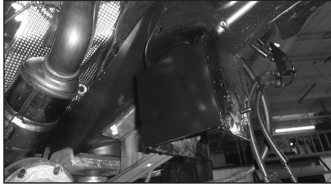
FIGURE 23 - SHOWN ALREADY PAINTED
