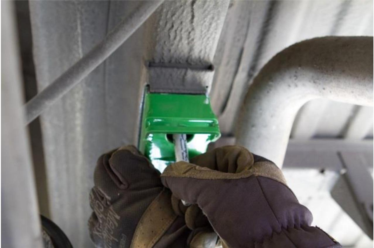
22) Since there is groove where the mounting holes land, a step drill will need to be used for drilling. Center punch the hole locations and drill with a step drill bit to a diameter of  $\frac{1}{4}$ " (7mm).
