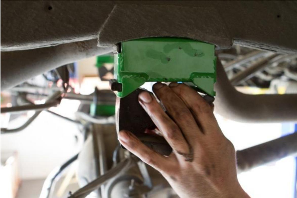
27) Once the second side is started, a screw driver, some wiggling and some additional lubricant will be needed to get the bump stop fully seated in the bracket.
