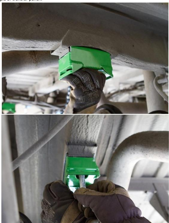
21) Since there is groove where the mounting holes land, a step drill will need to be used for drilling. Center punch the hole locations and drill with a step drill bit to a diameter of ¼" (7mm).
