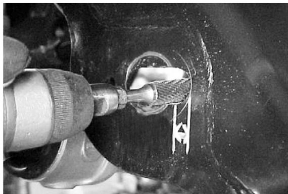
4. Remove any burrs after grinding and paint the exposed surfaces to prevent corrosion.
