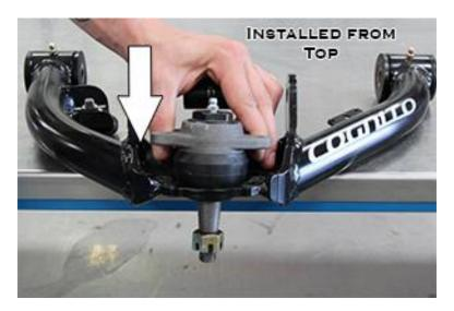
4. From the hardware package, insert the polyurethane bushings, crush sleeves, and grease fittings into the ends of the Upper control arms. Do not over tighten the grease fitting, tighten until it is snug. Use WD-40 to aid installation of bushings and use grease to aid installation of sleeves. See figure below.
