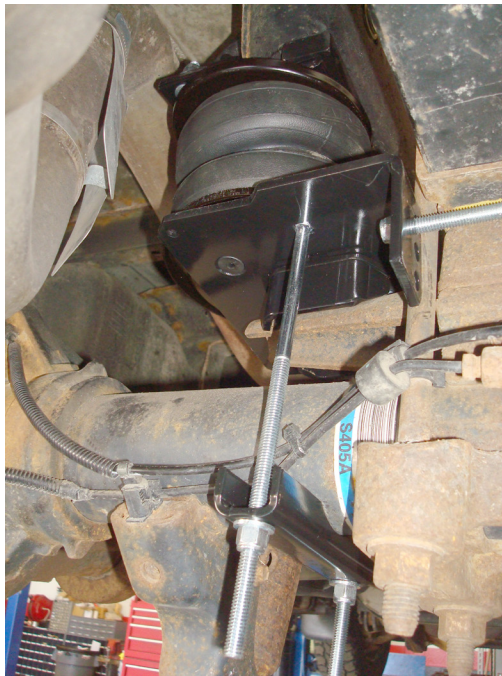
Back passenger's side (right) rear view of the kit installed.
